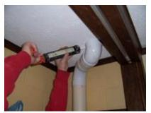
←You should have caulking installed around the vent pipe wherever it penetrates a wall or ceiling. If you have routed the ventilation up through an attached garage, fill both the
