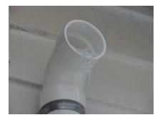
← Check to make sure there are no low spots or traps in the ventilation piping that could fill with moisture vapor condense.
