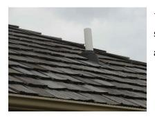
$\leftarrow In many cases, the outlet point will be above the roofline. If so, the outlet should end at a minimum height of 18 inches above the roof.$
