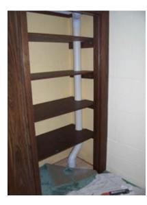
$\leftarrow$  The ventilation pipe is then extended up vertically to the floor joists. Once the ventilation pipe is up into or just beneath the floor joists, it is extended horizontally to the outside of the house or into an attached garage.
