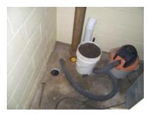
A radon mitigation system will collect and remove soil air below your basement floor from one of two sources:
