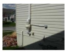
←A radon fan mounted on the outside of a house should be hard-wired into an electric circuit. If you mount a fan on the ventilation pipe in an attic, you can plug the fan into an outlet. For future reference, identify the electric circuit that powers the radon fan by labeling it in the electric panel box. Make sure to use brackets or hangers to secure the ventilation pipe to the house. Place the bracket or hanger every 72 inches horizontally and every 96 inches vertically. $\rightarrow$
