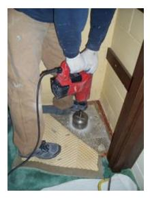
←If your home does not have a sump pit, then a five-inch diameter suction hole will be drilled through the basement floor. This suction point is typically installed in a furnace or utility room in the basement about one to two feet in from an outside wall.
