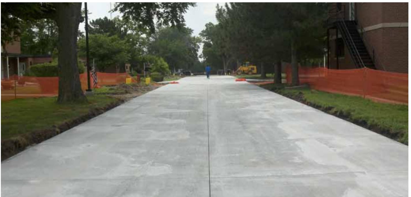
A new 525-foot stretch of road, Daily Drive, at YRTC-K.
