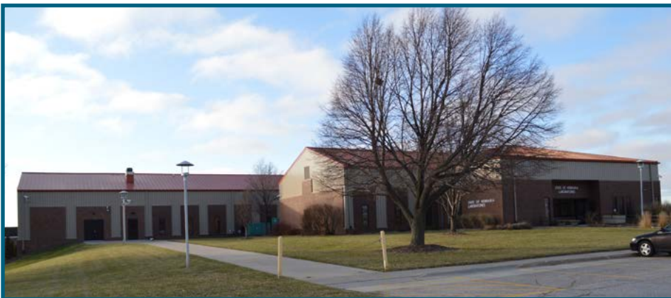
The building that houses the Nebraska Public Health Environmental Laboratory was built in the mid-1970s on the southwest edge of Lincoln, Nebraska.
